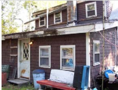
Sagging Roofs, Detached Gutters
