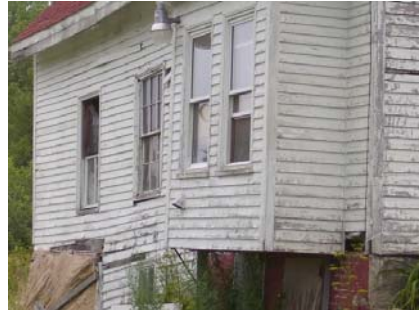
Sagging Walls, Cracked and Missing Foundation
