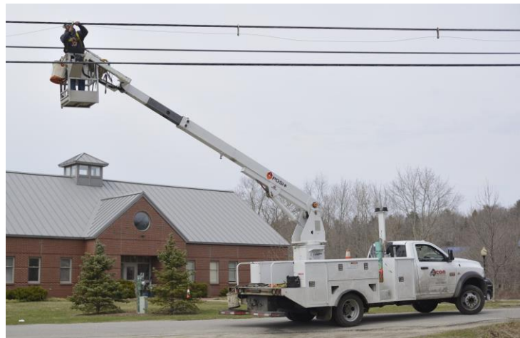
Figure 2: Construction worker lashes fiber to poles in Rockport.
